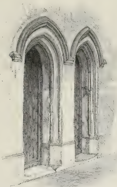
Fig. 30. Double Doorway on the west side of the Cloister.
